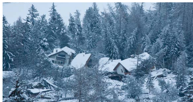
On-site inspection of the emergency forces in the hours after the slide in the abbey; damages to residential houses in the hamlet of Sottrù (Municipality of Abtei, South Tyrol, Italy)
